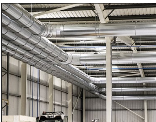
Multiple duct runs designed for optimum energy efficiency.
