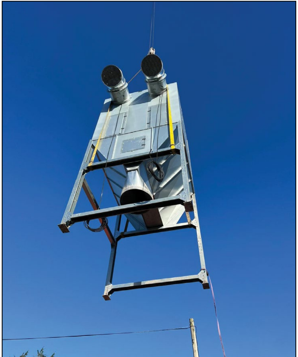
Dropping into place: the new Wood Waste Control dust extraction filter is hoisted on to site at West Sussex Office Furniture.
