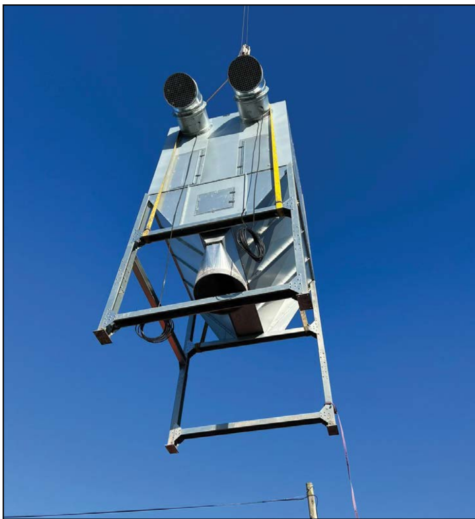
Dropping into place: the new Wood Waste Control dust extraction filter is hoisted on to site at West Sussex Office Furniture.
